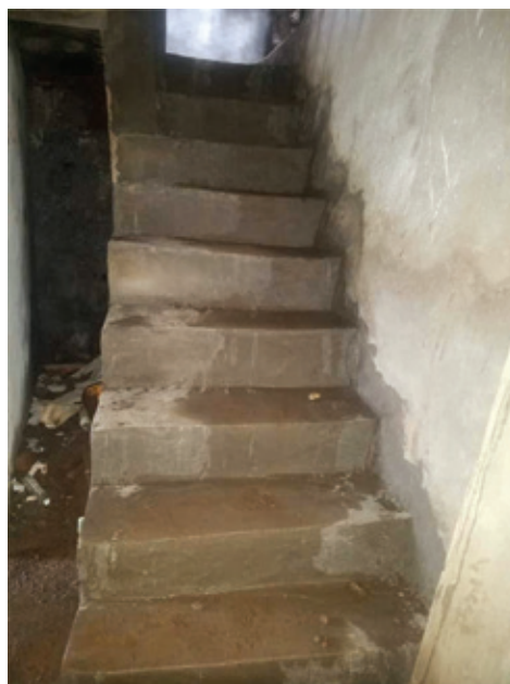
Security gates were installed to protect the students and property. The lower level stairwell steps were rebuilt and the walls were white washed to brighten the stairwell.
